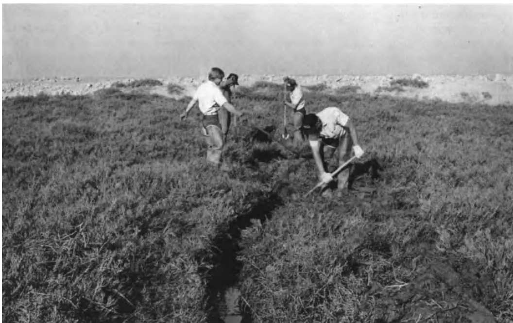
Figure 14.1. Using hand labor for ditch maintenance for management of saltmarsh mosquitoes (photograph by John R. Rusmisl, courtesy of Alameda County Mosquito Abatement District).
